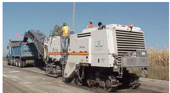
Milling machine milling asphalt road and loading debris into haul truck.
