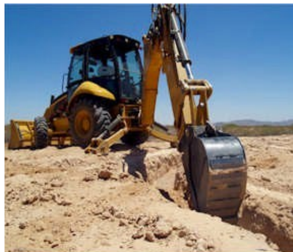
Backhoe with enclosed cab.
