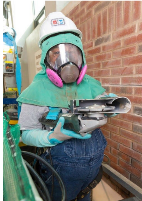
Worker is showing a handheld grinder equipped with shroud.
