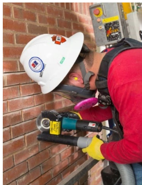
Worker grinding mortar from between bricks (tuckpointing) with a handheld grinder equipped with a shroud and dust collection system using respiratory protection.
