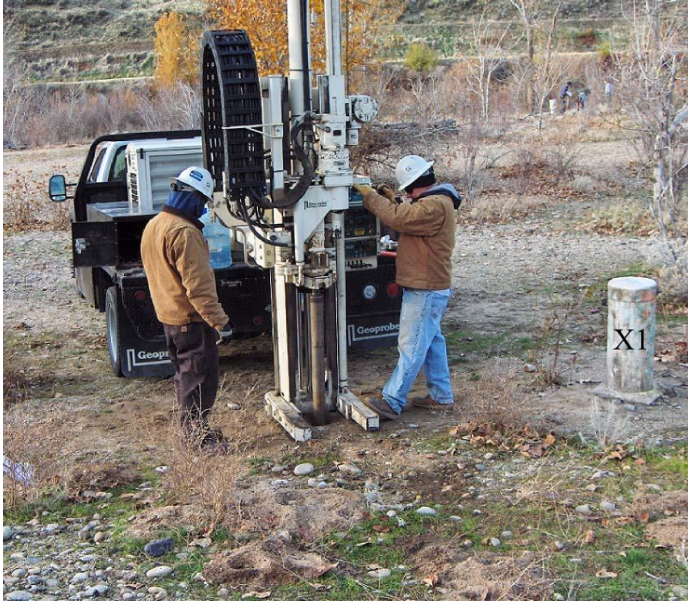
Figure 3: Installation of neutron access tube NX1 using Geoprobe direct push equipment.
